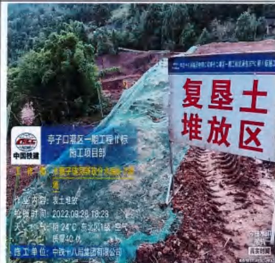
总干 6-7 渣场表土堆放及防护
